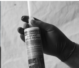
#3 Hold cartridge upright and screw on mix tube.
